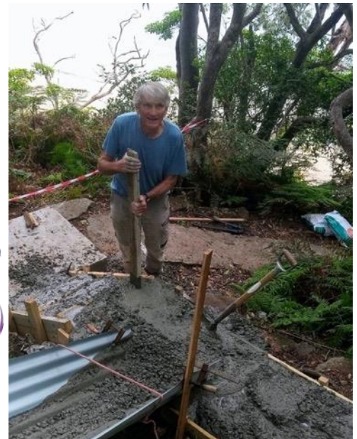
The indefatigable Bruce Davis repairs the Davis Marina path which he helped to build when he was a cabin boy with the First Fleet.
